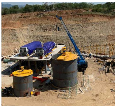
Filter Press Construction
